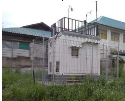
Gambar 13. Foto Air Quality Monitoring System di Mako Satpol PP Batam
