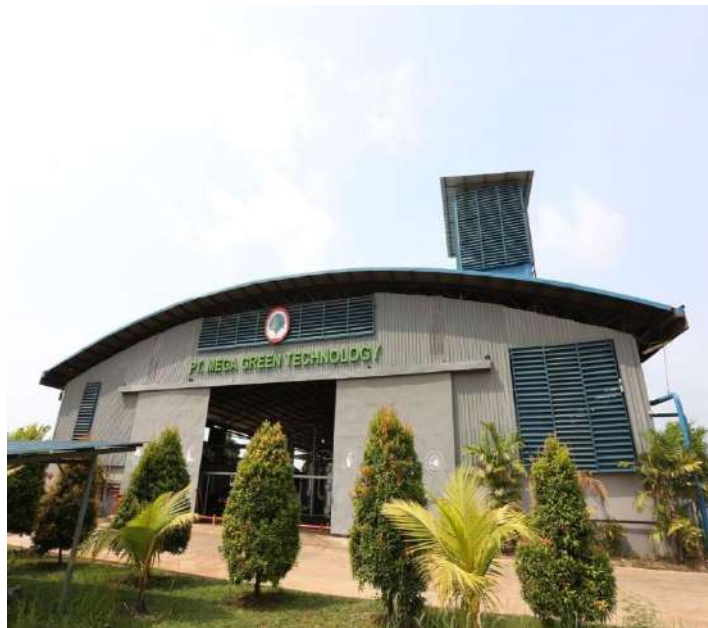
Gambar 4.14 Gedung PT Mega Green Technology
